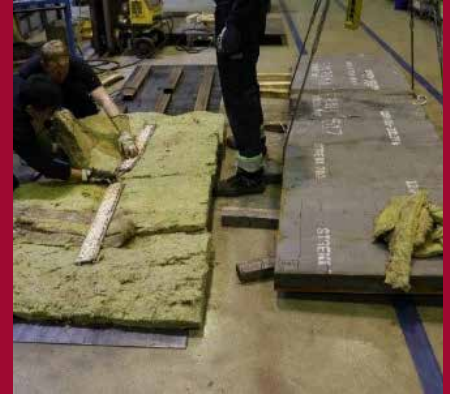
3. Cover it with insulation
